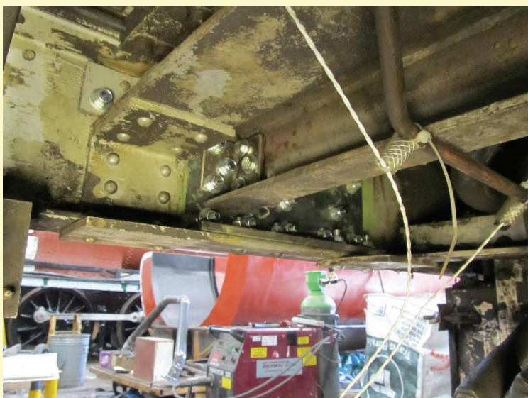
The sole bar repair plate, 15/4/13
