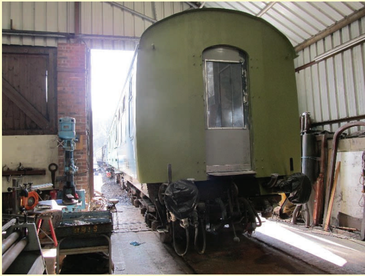
51566's corridor end repairs, 20/4/13
